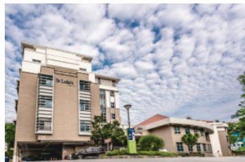
St Luke's Hospital (SLH)
